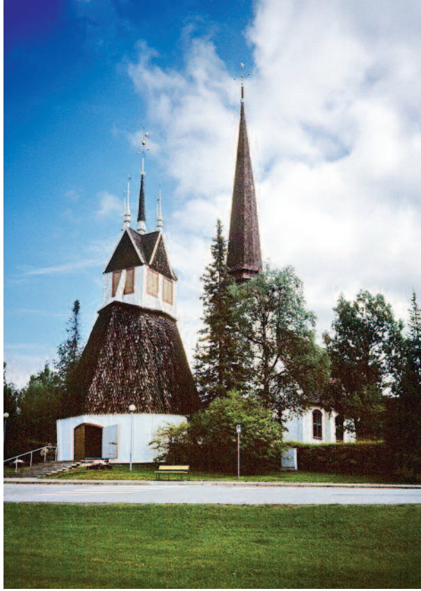
Figure 5-1. Torneå (Tornio) church close to the Arctic circle, southern end point in 1736 of the French arc measurement, led by Maupertuis.
